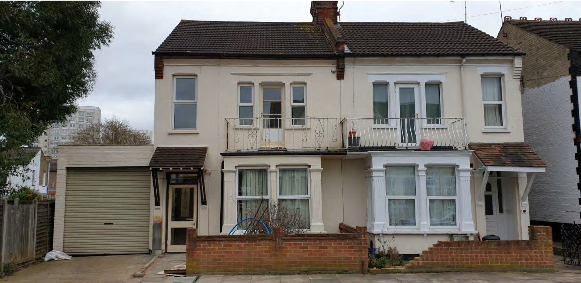
Front elevation during refurbishment, 2019
