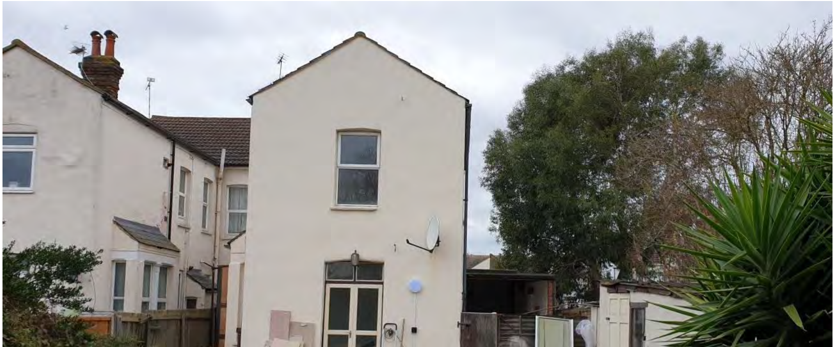
Rear elevation of site during refurbishment in 2019
